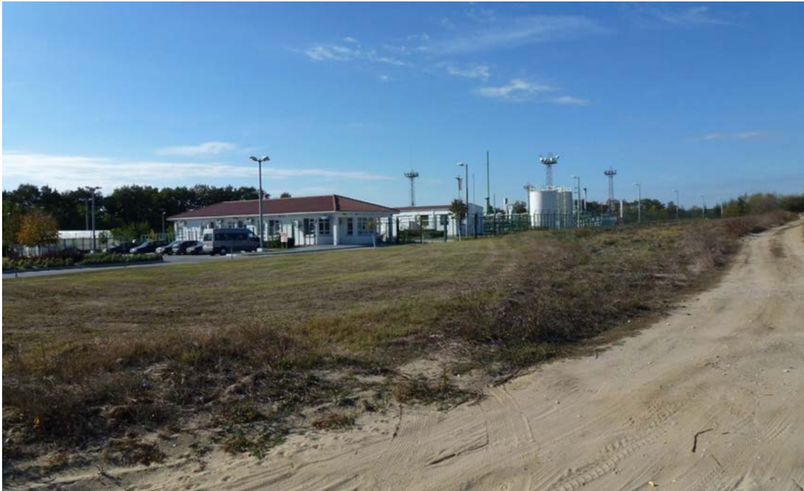
Figure 5.11b: Galata Gas Processing Plant
