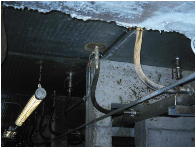
Figure 10: Example of biogas blowing from bottom of a Valorga fermenter (left) and a mechanical low speed mixer (right)
