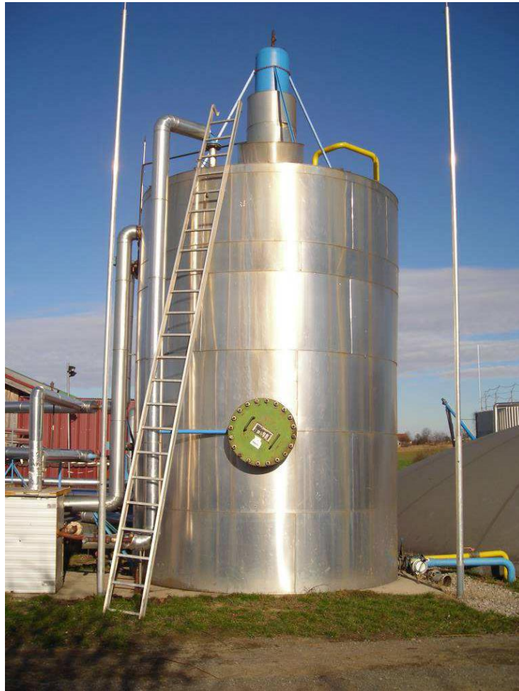
Figure 8: Example of pasteurisation unit (Source: Bios1 GmbH)
