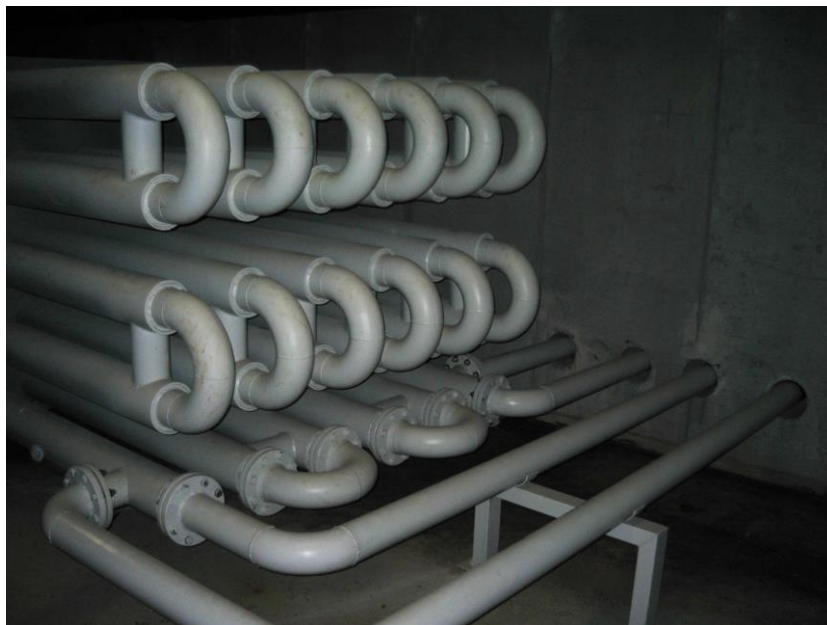
Figure 11: Example of heat exchanger for ingestate pre-heating
