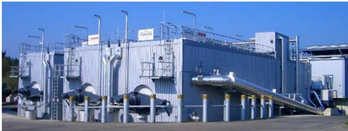
Figure 3: Horizontal, dry digestion system (Source: Kompogas)
