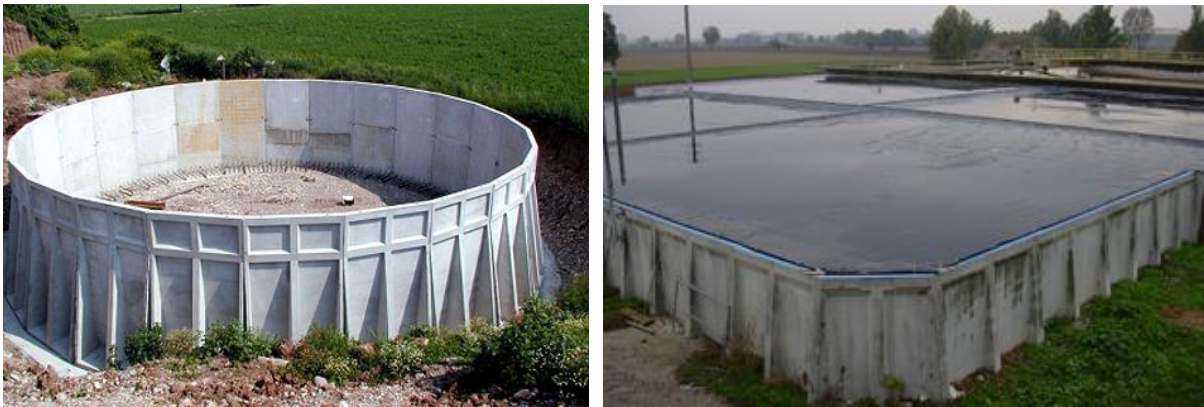
Figure 16: Example of a uncovered (left) and covered (right) digestate storage tanks
