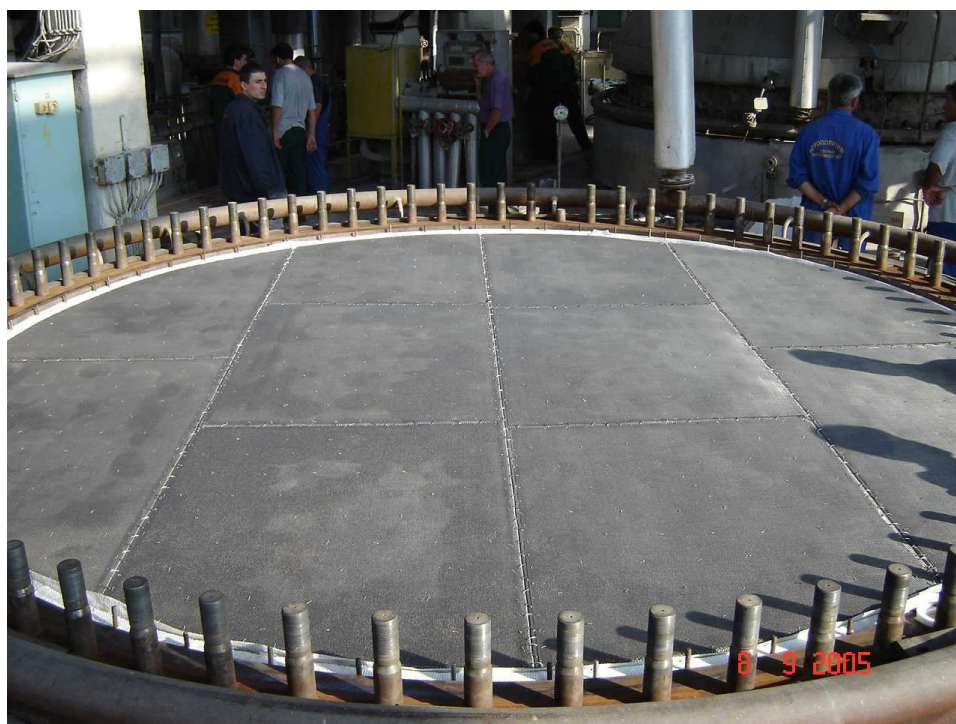
Figure 6 Installing of the catalyst for converting N_2O
