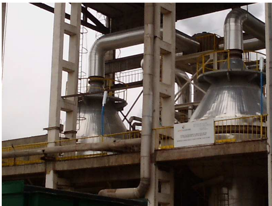
Figure 5 Photo of two of the four reactors ( \text{NH}_3 burners)
