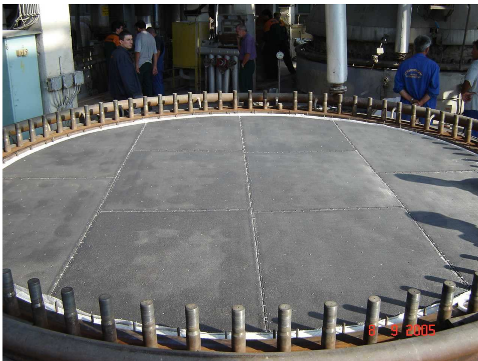
Figure 6 Installing of the catalyst for converting N_2O
