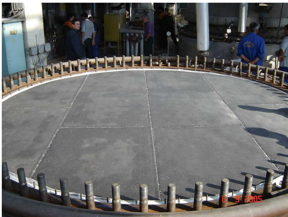
Figure 6 Installing of the catalyst for converting N_2O
