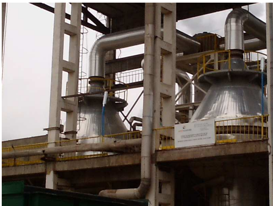
Figure 5 Photo of two of the four reactors (NH 3 burners)
