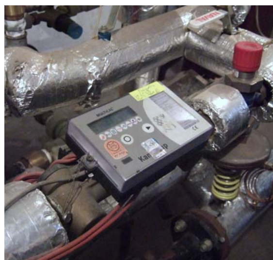
Photo-9 Heat meter in the Sub-station
