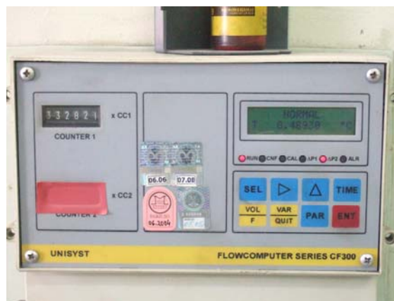
Photo-12 Heat meter of Zemlyane HP
