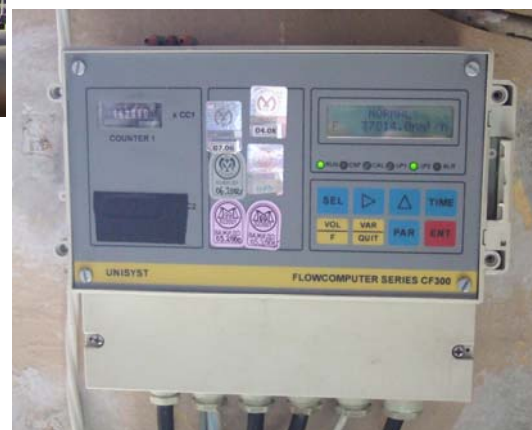
Photo-7 Gas flow meter for boiler in Sofia CHP
