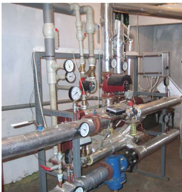
Photo-8 Heat supply Sub-station in the residential apartment house
