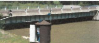
Figure 1.2.1 Gauge with wooden shelter, solar panels, satellite antenna, and one weight gauge on bridge
