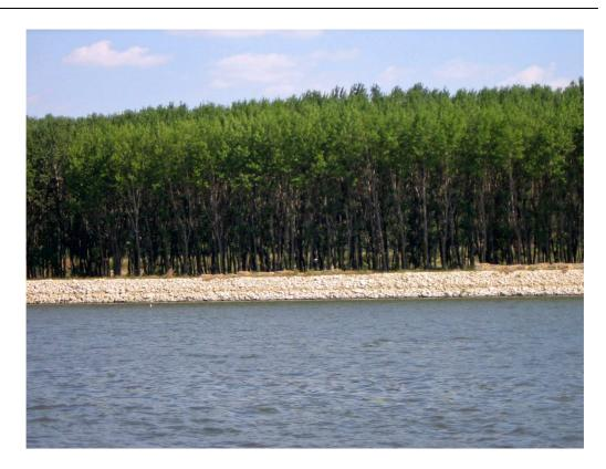
Figure III-5: Right bank protection at rkm 536
