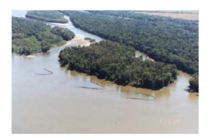
Figure 5.12: Chevron structures Carroll Island, USA (Source:US Corps of Engineers, 2008)
